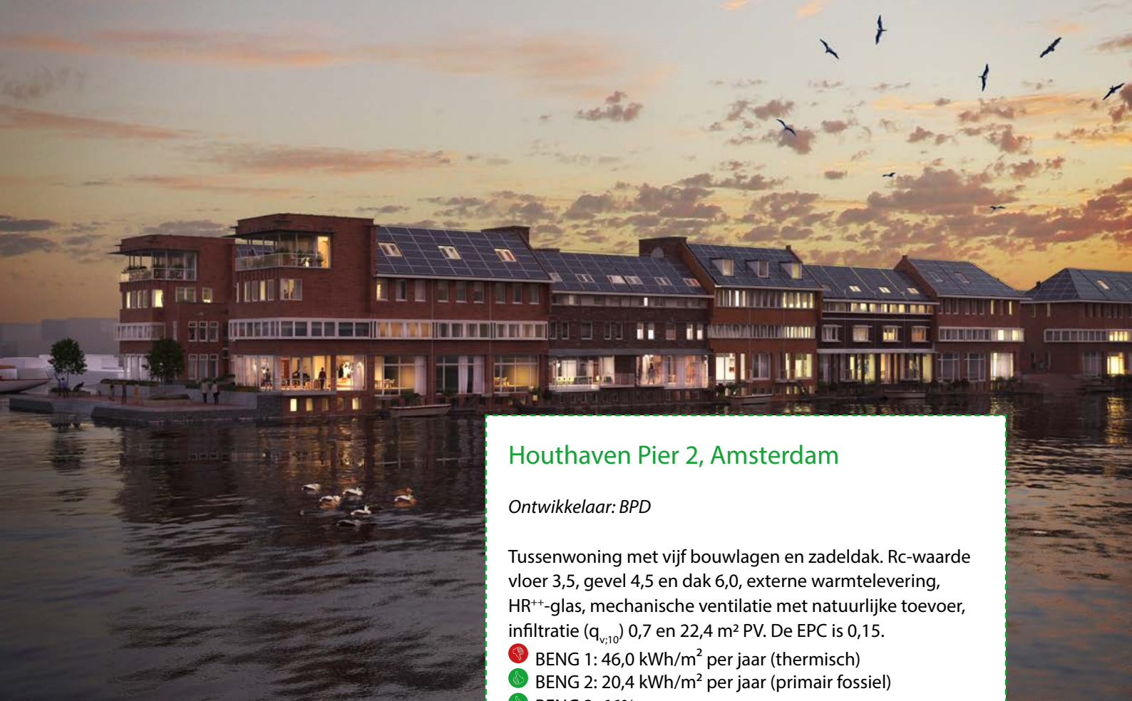
Houthaven Pier 2 Amsterdam (BPD)
